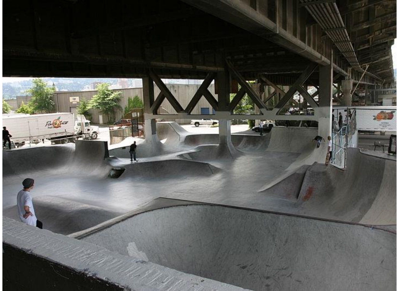
Image Credit: "Utilizing the Space Beneath Bridges" streets.mn
